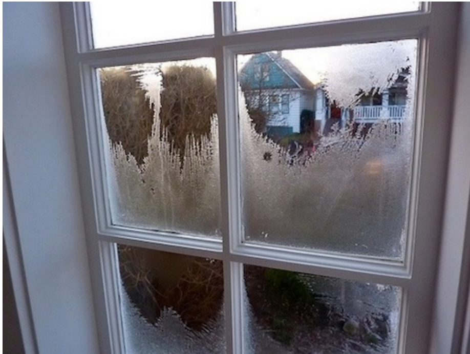
Frost formation on interior surfaces
