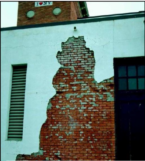
Freeze-thaw damage
