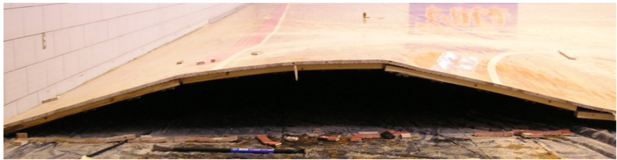
Wood deformation: Shrinking, swelling
