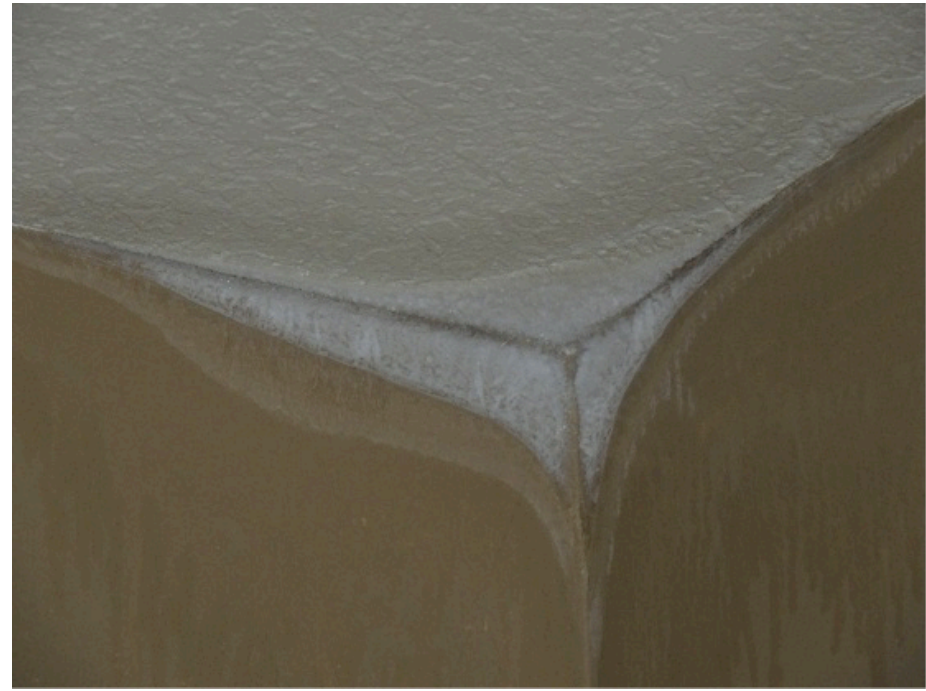
Frost formation on interior surfaces
