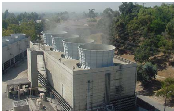
Water-cooled chiller (w/ cooling tower – larger capacity & more efficient)
