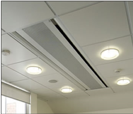
Chilled beams
