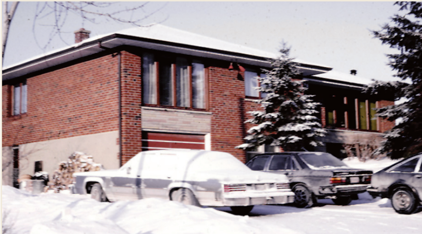
PHOTO 1 Mom and Dad's House. Small house in Downsview, ON, Canada, with triple-glazed casement windows and a super-insulated vented attic with an airtight ceiling.
