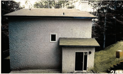
PHOTO 7 More Earth Tubes. Note the small wood box off to the side of the house on the hill. That is the intake location for the earth tubes. I got an award for what is probably the ugliest house ever built in Ontario. There is a reason we don't let engineers do architecture. Yes, that is the only window on the north side. No windows on the east and west. Lots of windows on the south.
