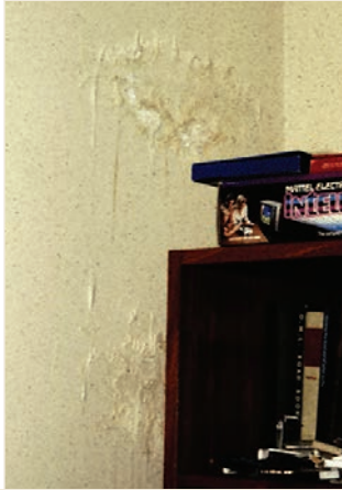
PHOTO 3 (LEFT) My Room. The condensate began to leach through the exterior wall to the interior and damage the plaster. But no one could see it because it was occurring behind a bookcase. This was occurring in my old room. My room. Not my brother's old room. My room. PHOTO 4 (CENTER) Signs of Spillage. The telltale soot markings indicative of spillage and backdrafting of products of combustion. PHOTO 5 (RIGHT) Flue Liner. Warming the chimney using a flue liner to reduce the size of the flue and reduce the heat loss through the chimney. This increased the temperature of the flue gases and the theoretical draft.
