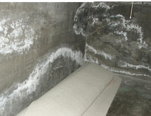
Efflorescence
