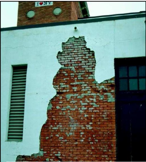
Freeze-thaw damage
